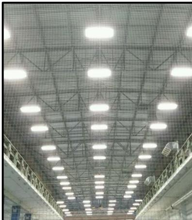
Figure 8: LED replacement lights installed in a high bay facility.
