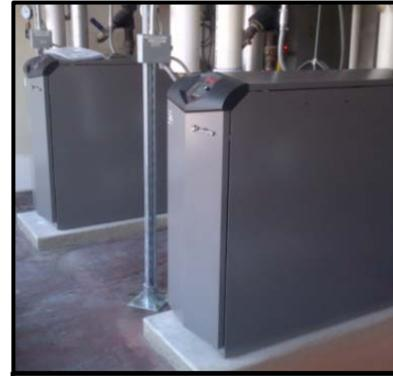
Figure 7: High efficiency boiler units that replaced central steam.
